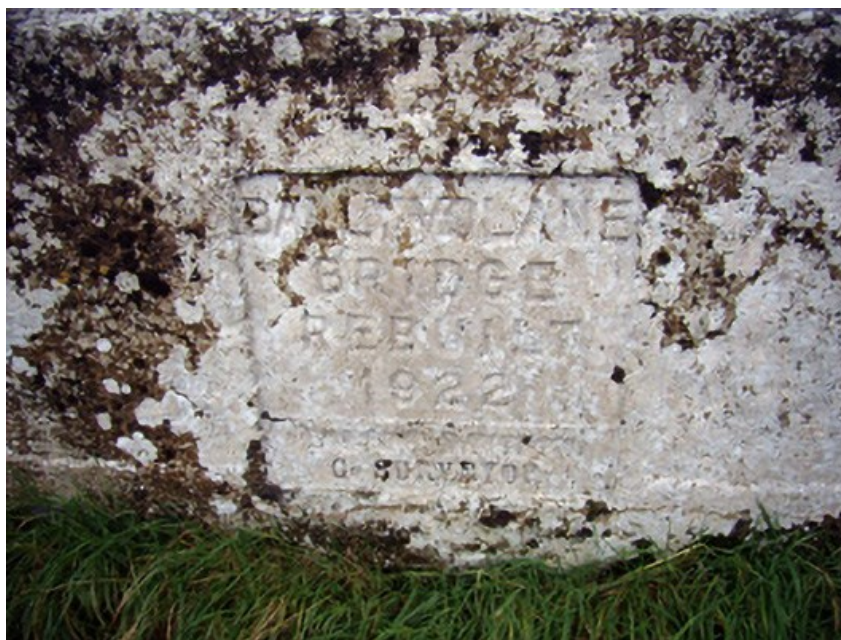
Figure 3: Ballyvolane Bridge, sign showing rebuilt in 1922 date:
